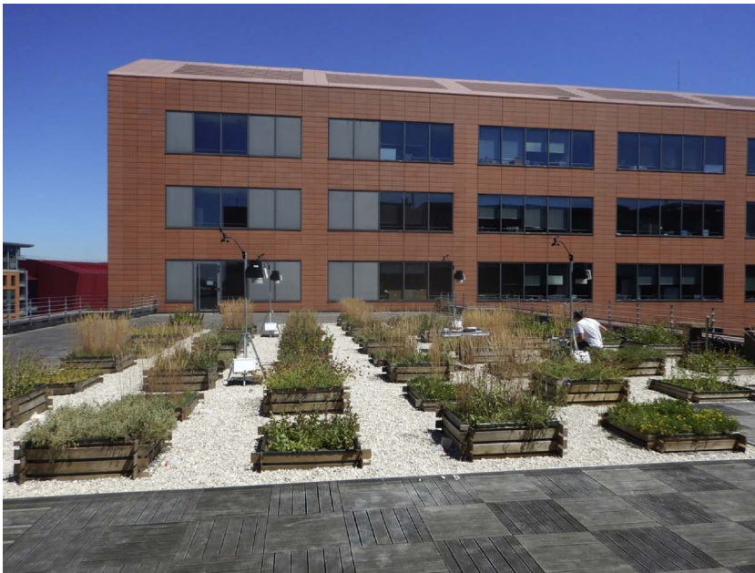
Fig. 1. Experimental green roof in Paris City, France, manipulating substrate type, substrate depth and plant diversity © Yann Dusza 2016.
